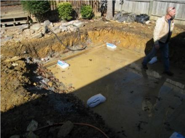
Figure 7. Ice Bag Positioning in Excavation
